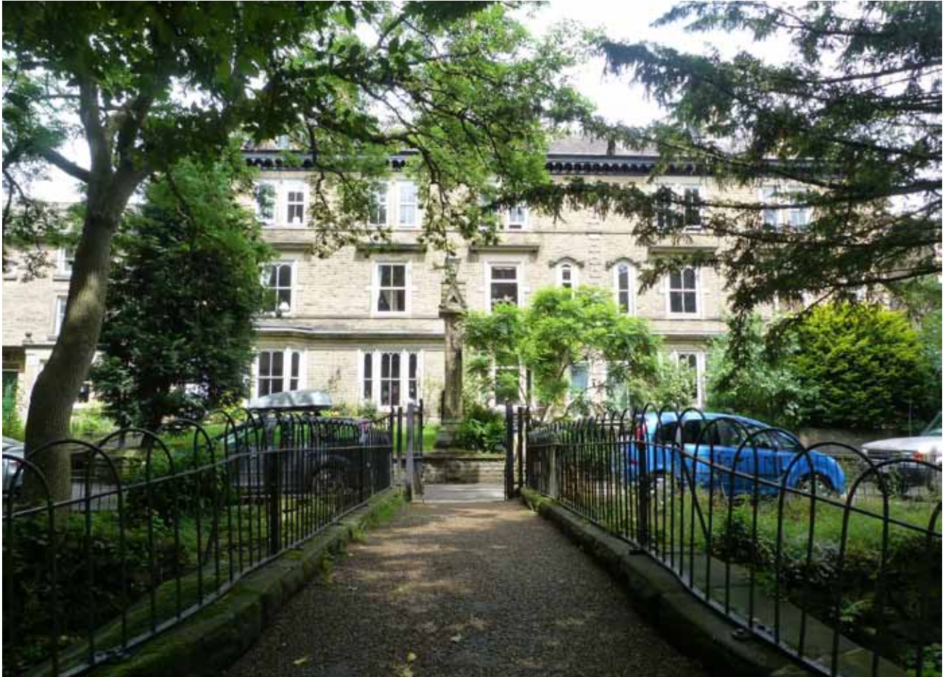
Knowleston Place, Matlock
